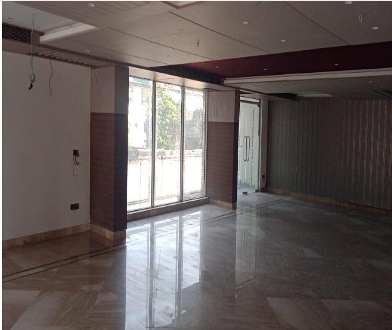
Club House : Banquet Hall Flooring , False Ceiling , Wall Panelling and Electrical Works
