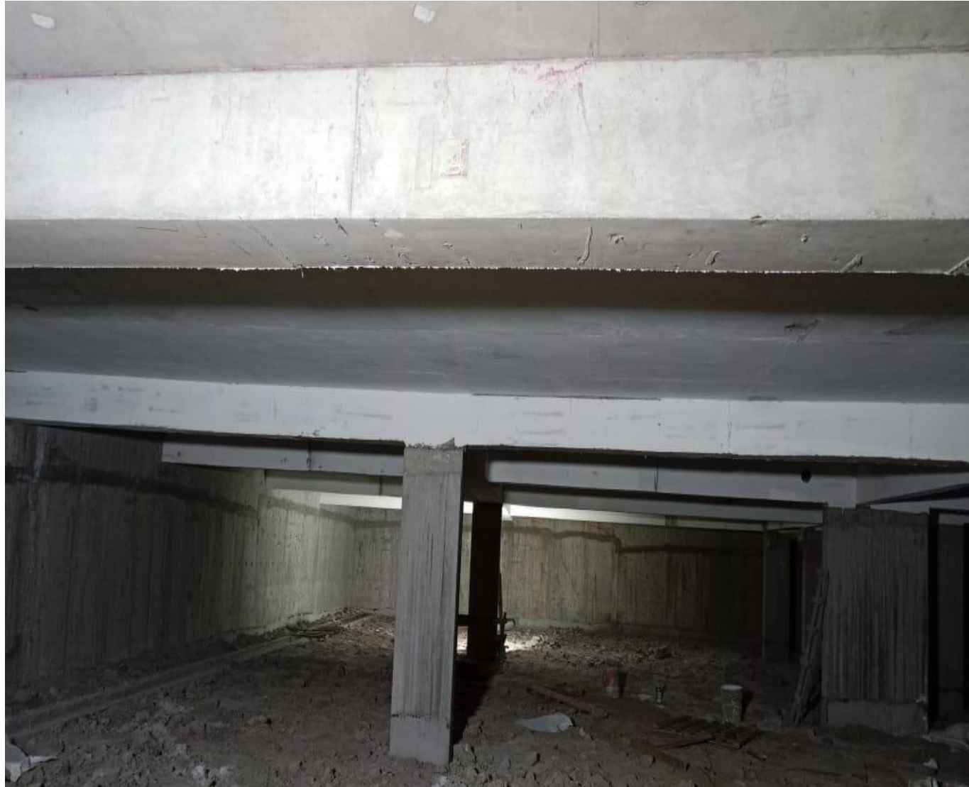
Basement: Filling Work
