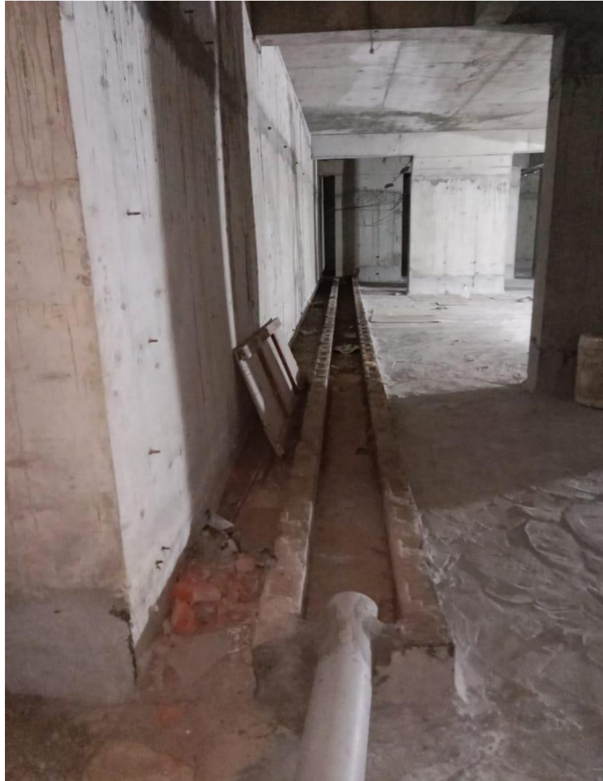
Basement: Drainage Work
